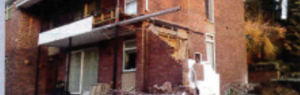
Demolishing the single storey side wing
